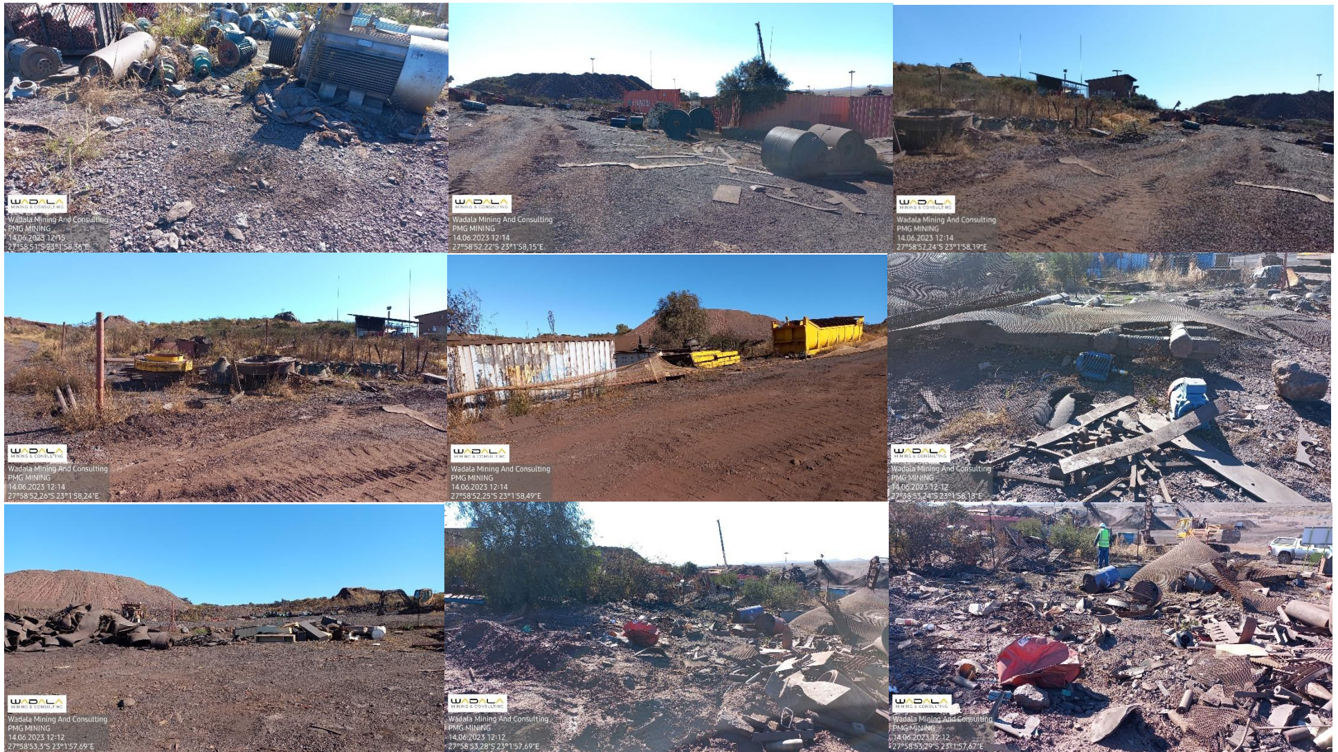
Photo 14a: Salvage yard/ Laydown area at Processing Plant
