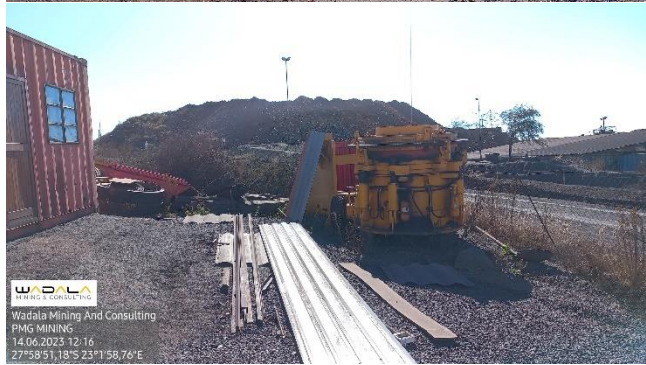
Photo 14b: Salvage yard/ Laydown area at Processing Plant
