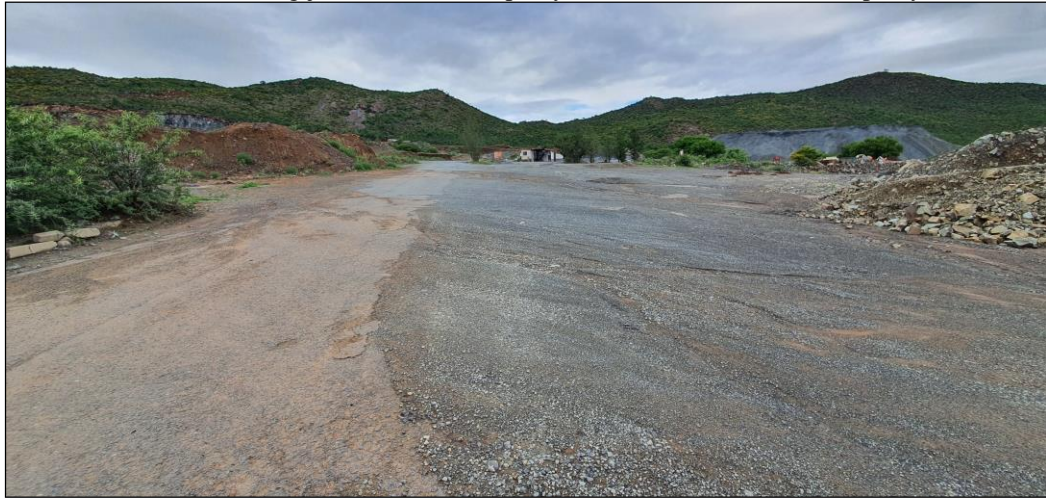
Figure 10: General view of one of the access roads to the quarry
