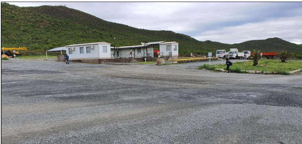
Figure 12: General view of the offices and associated infrastructure
