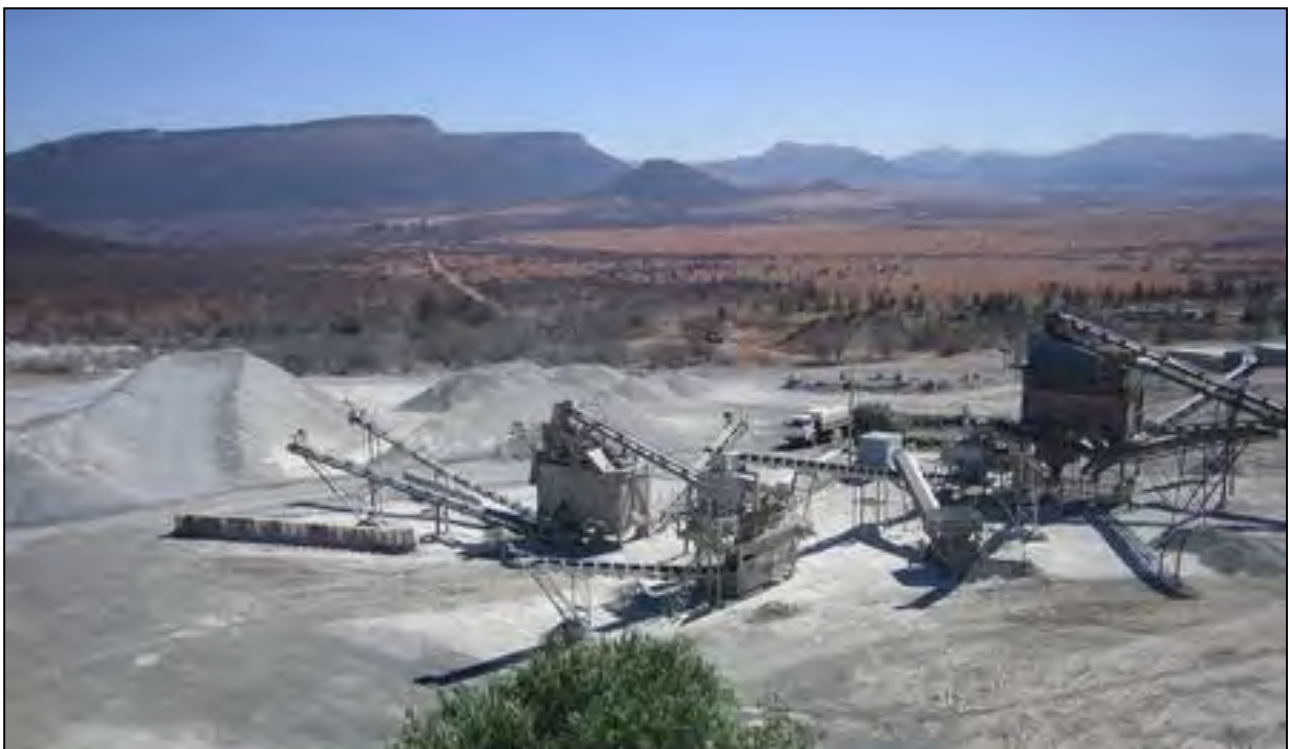
Figure 6: Photograph of stockpiles and plant area
