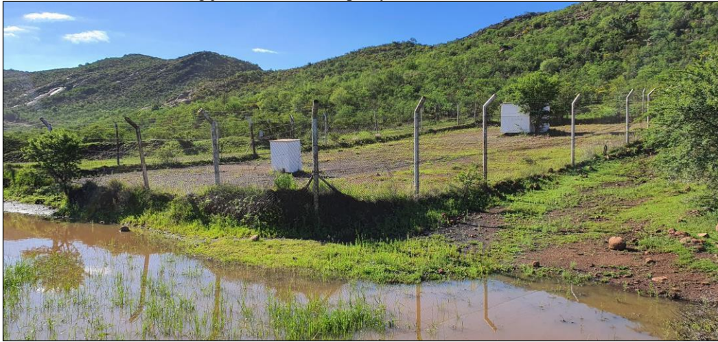
Figure 25: General view of the eastern slopes of the survey footprint (access roads)
