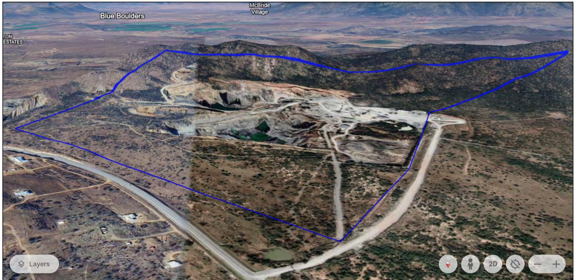
Figure 12: Google Earth 3D view (from the north) of the topography of the site (Queenstown Quarry).
