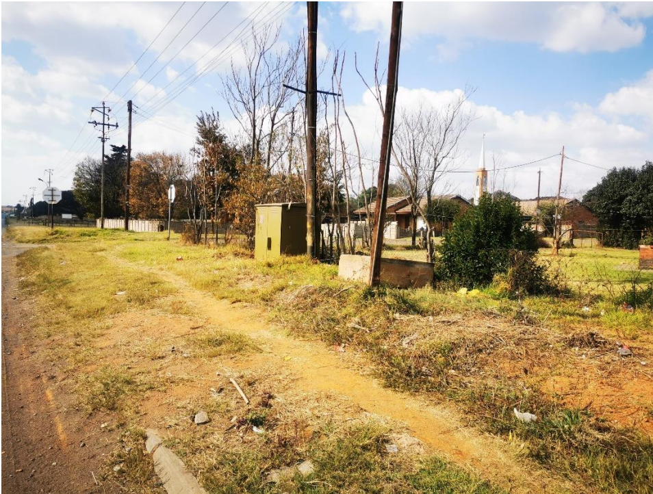
Figure 8-17 Electricity distribution lines and transformer
