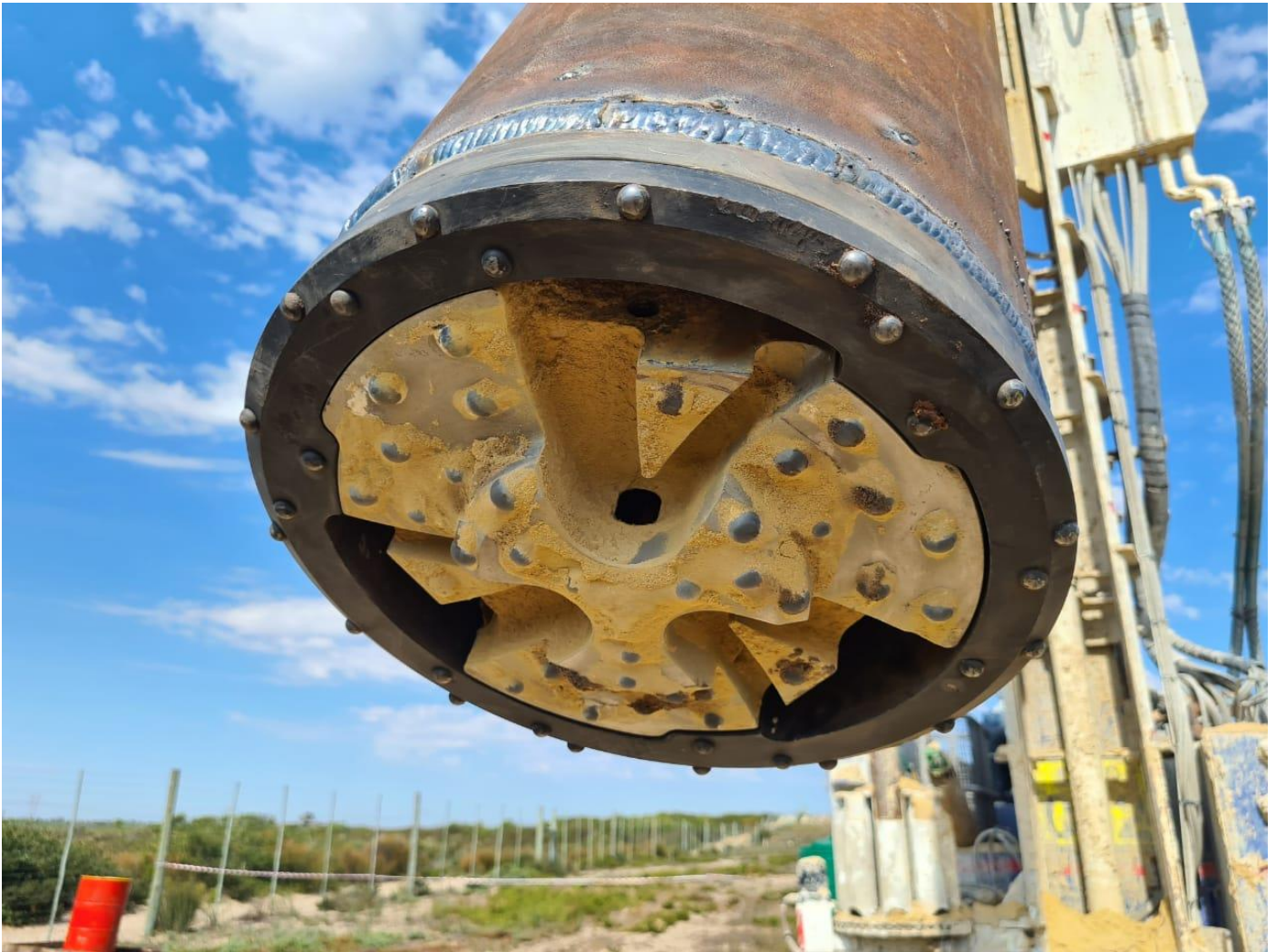
Figure 6-3: Large diameter drilling for rescue boreholes (Georoc, 2024)
