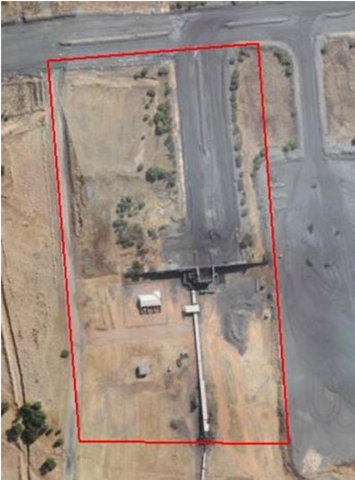
Figure 6-7: ROM conveyor tip area
