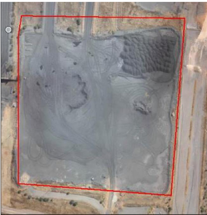
Figure 6-8: Emergency ROM stockpile area
