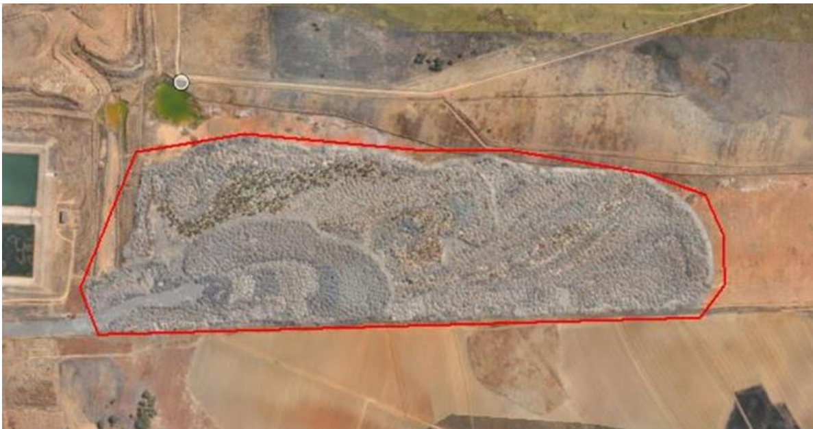
Figure 6-11: PCD1 overburden stockpile
