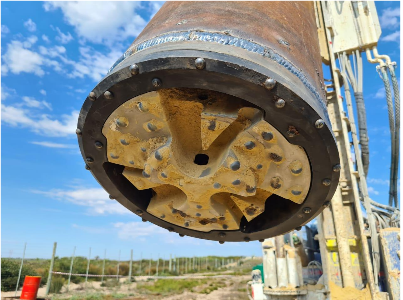
Figure 5-45: Large diameter drilling for rescue boreholes (Georoc, 2024)
