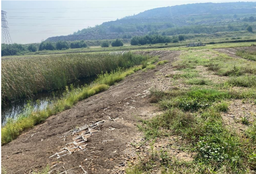
Photo 1: Wall crest condition
