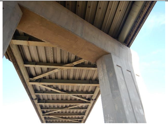
Fig. 3.18: Concrete pier cap
