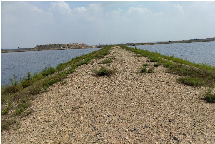
Photo 1: Wall crest condition
