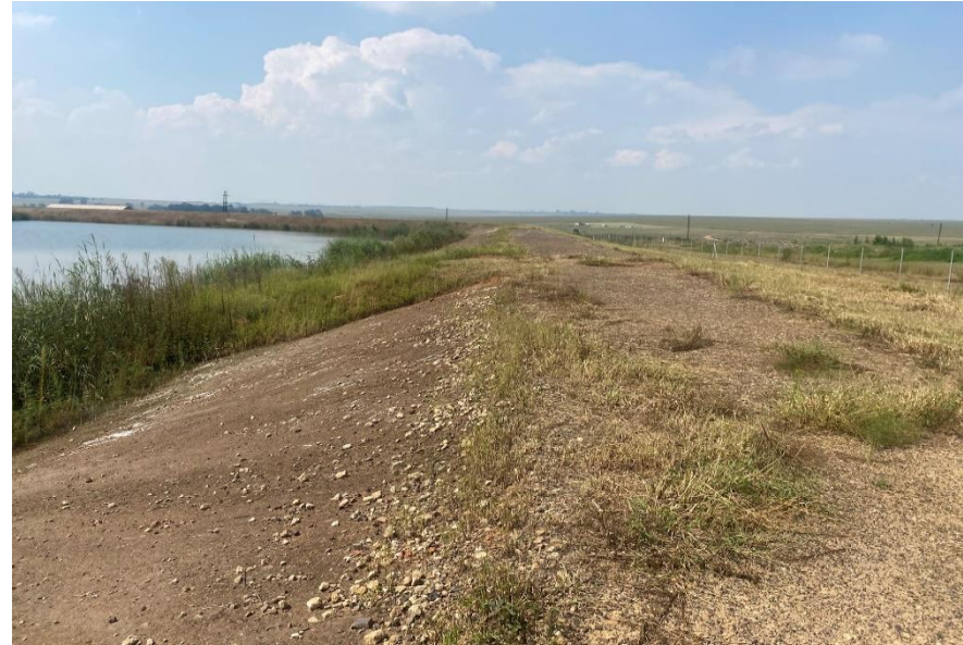
Photo 2: Wall crest condition
