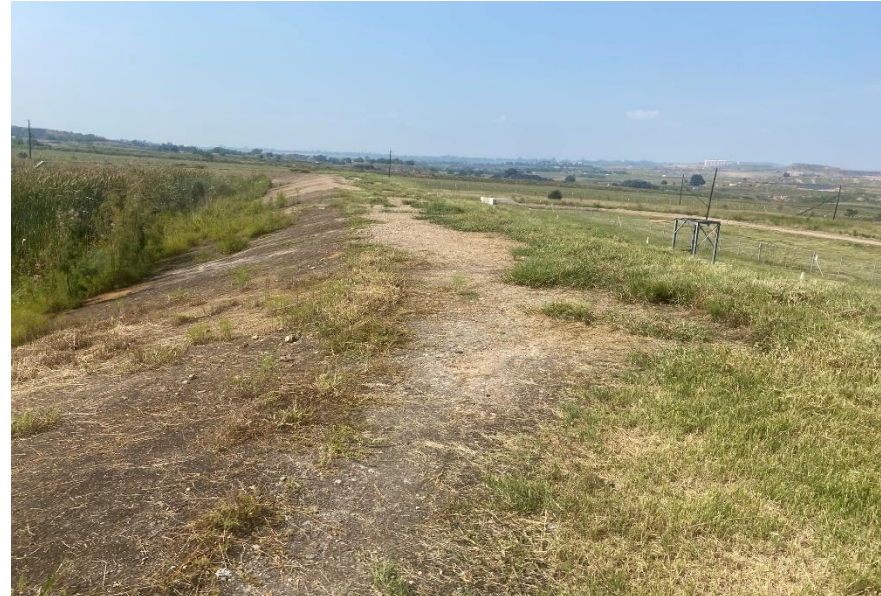
Photo 2: Wall crest condition
