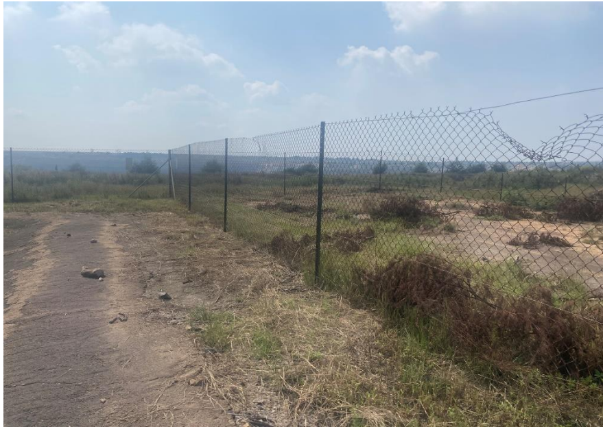
Photo 1: Wall crest condition
