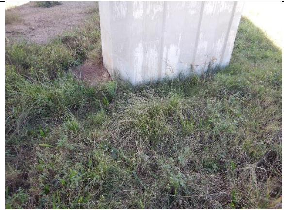
Fig.3.16: Base of the concrete pier
