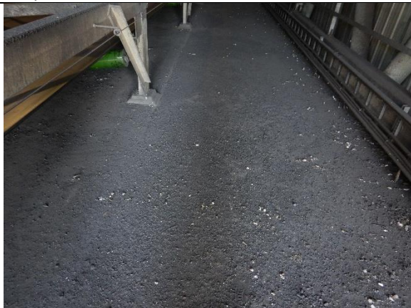
Fig. 3.23: Surface of the deck
