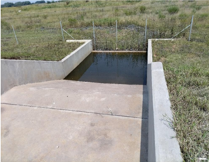
Photo 11: Outflow spillway
