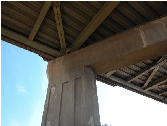
Fig. 3.15: Concrete pier cap
