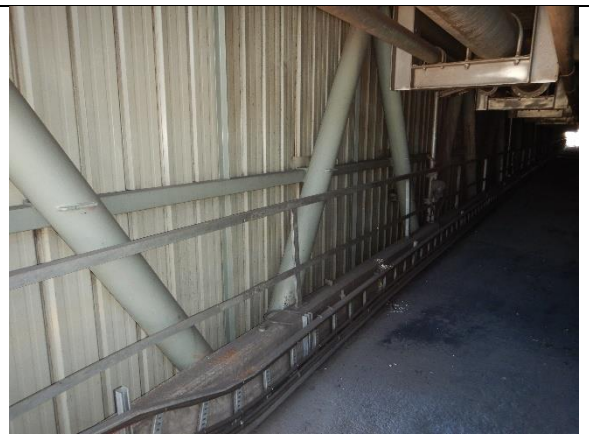
Fig. 3.20: Internal cladding sheets and side bracing assemblies
