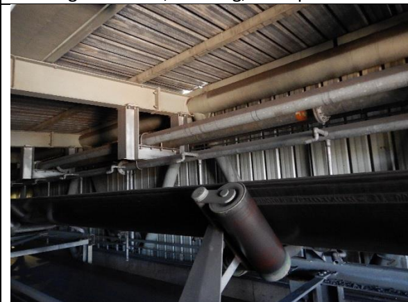
Fig. 3.19: Interior of the enclosed walkway structure
