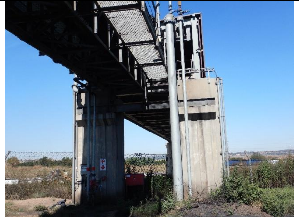
Fig. 3.10: Bridge support piers
