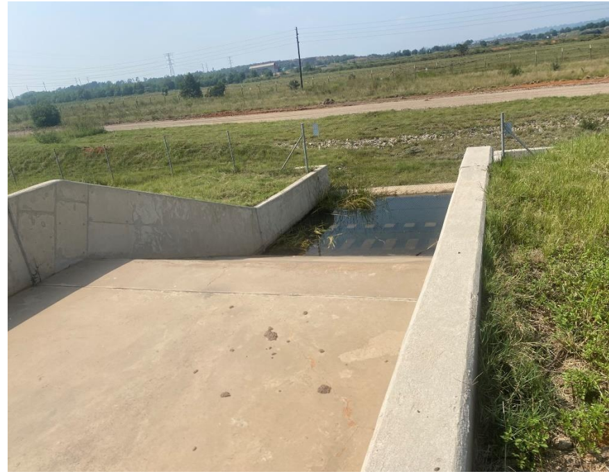
Photo 12: Outflow spillway
