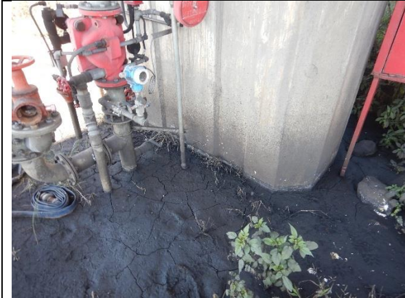
Fig.3.9: Base of the concrete pier
