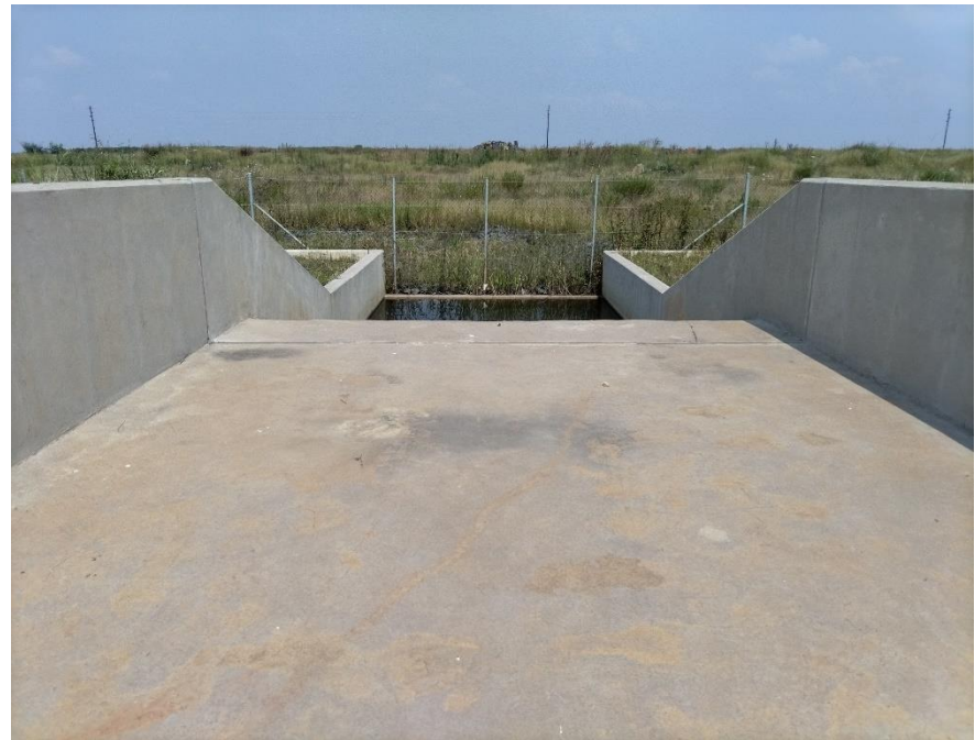
Photo 12: Outflow spillway
