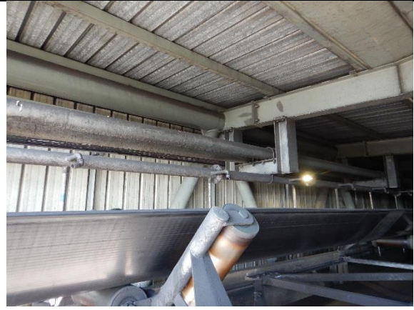
Fig. 3.22: Interior of the enclosed walkway structure
