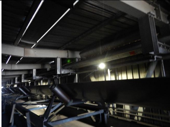
Fig. 3.21: Interior of the enclosed walkway structure
