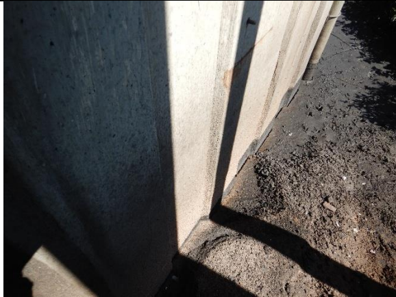
Fig.3.5: Base of the concrete pier
