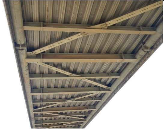
Fig. 3.14: Floor beams and cross bracing
