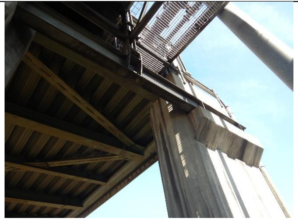
Fig.3.2: Steel floor beam girders
