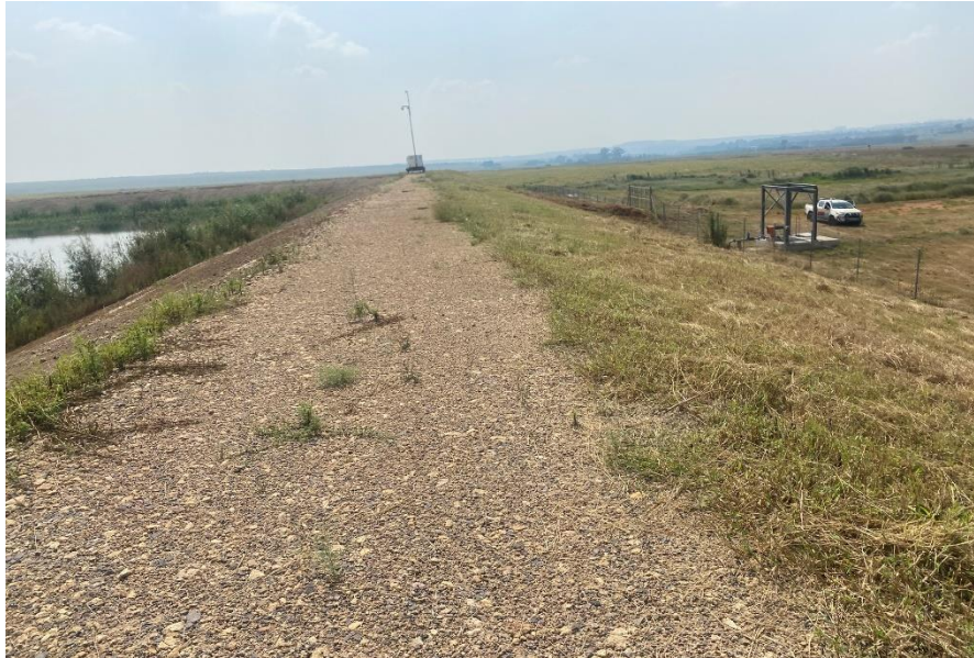
Photo 1: Wall crest condition
