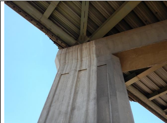
Fig. 3.17: Concrete pier cap
