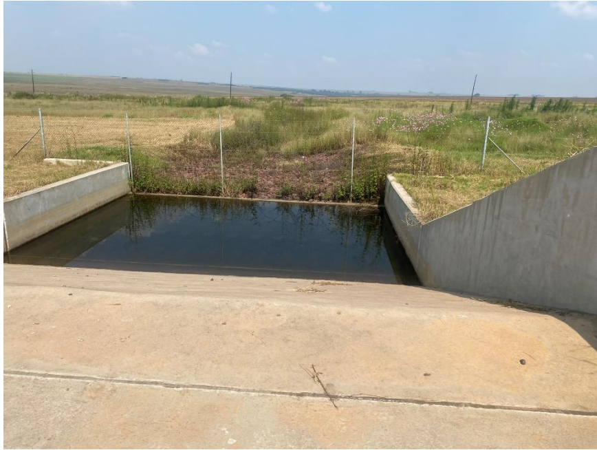
Photo 13: Overflow spillway
