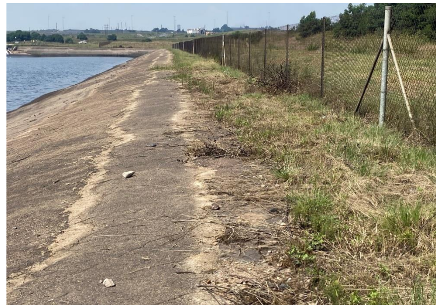
Photo 2: Wall crest condition
